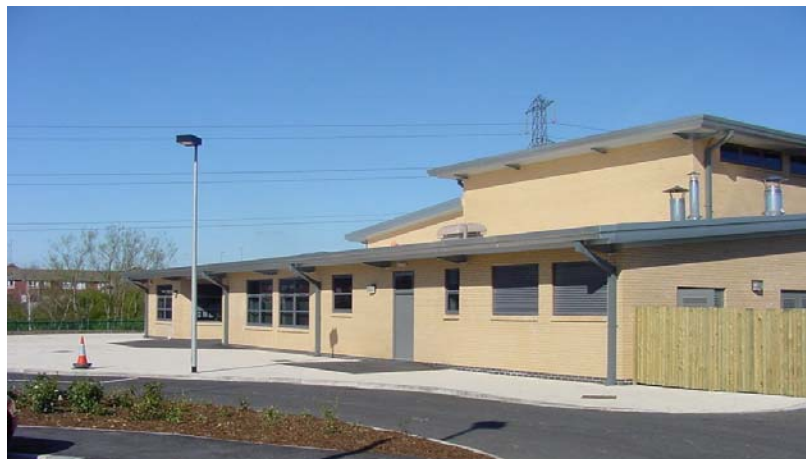
Arundale Primary School, Hattersley (PFI), Opened September 2002
